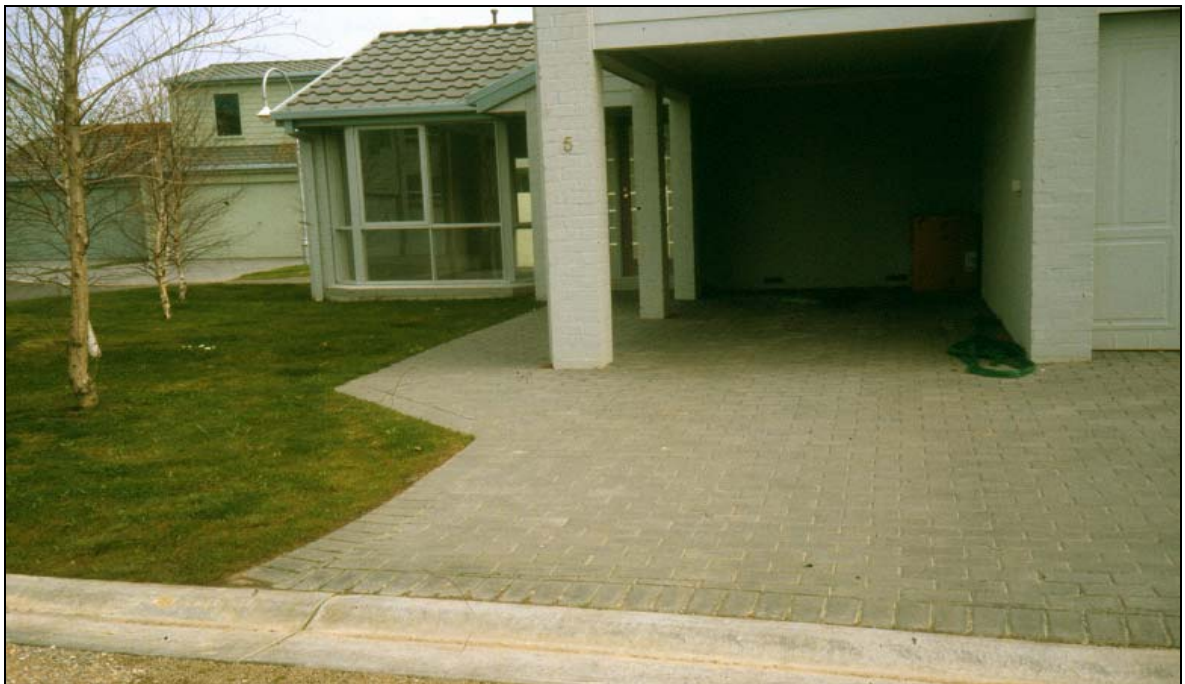
Figure 4: Undifferentiated paving of driveway and entry pathway limit dwelling individuality
