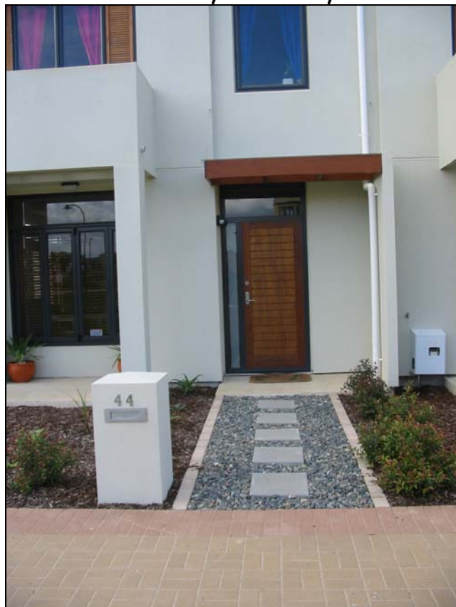
Figure 28: This bare entry and awkward path in new medium-density housing in Auckland, NZ do not communicate 'welcome'
