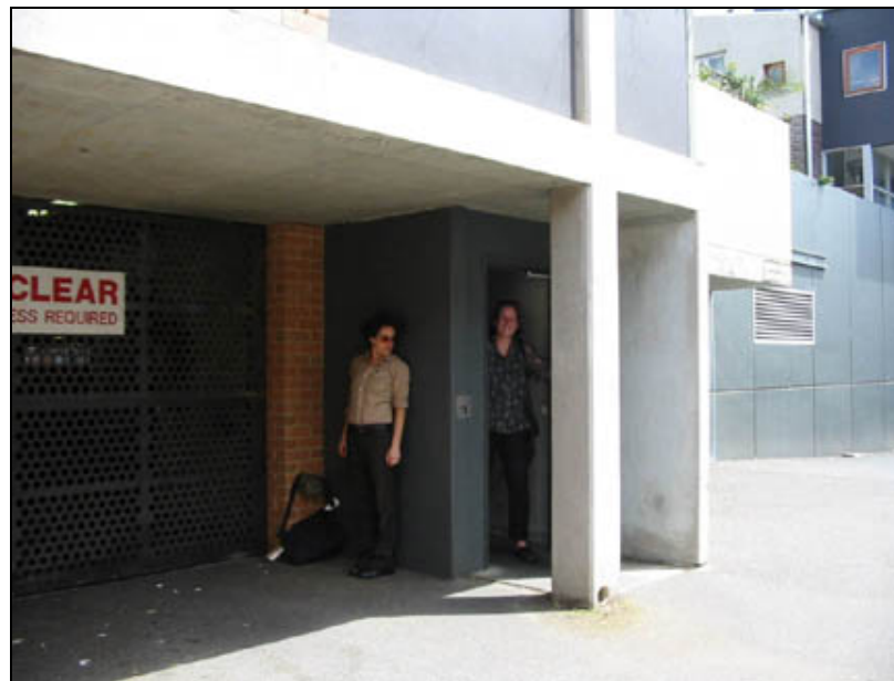
Figure 9: Entrapment area at building entry
