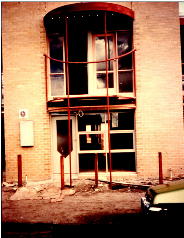
Figure 5: Natural Ladder A
