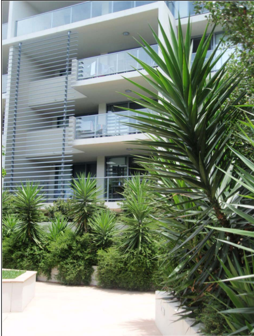
Figure 17: 'Natural ladders' diminish the security of balconies
